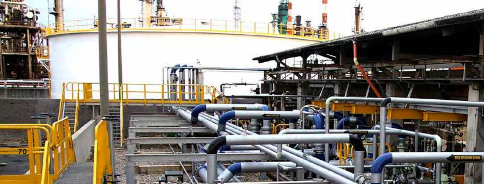
Pumping House Barrancabermeja Refinery, Santander department
