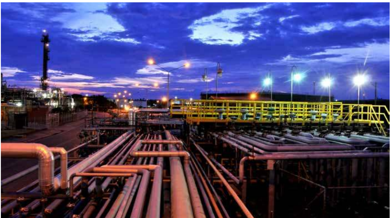
Barrancabermeja refinery, Santander department
