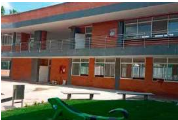
Construction phase II La Fortuna school
